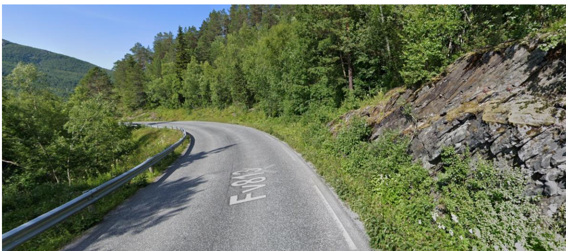
Figur 2-12: Bergskjæring, ca. P900.
