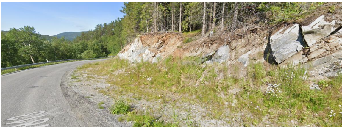
Figur 2-13: Bergskjæring, ca. P1050.
