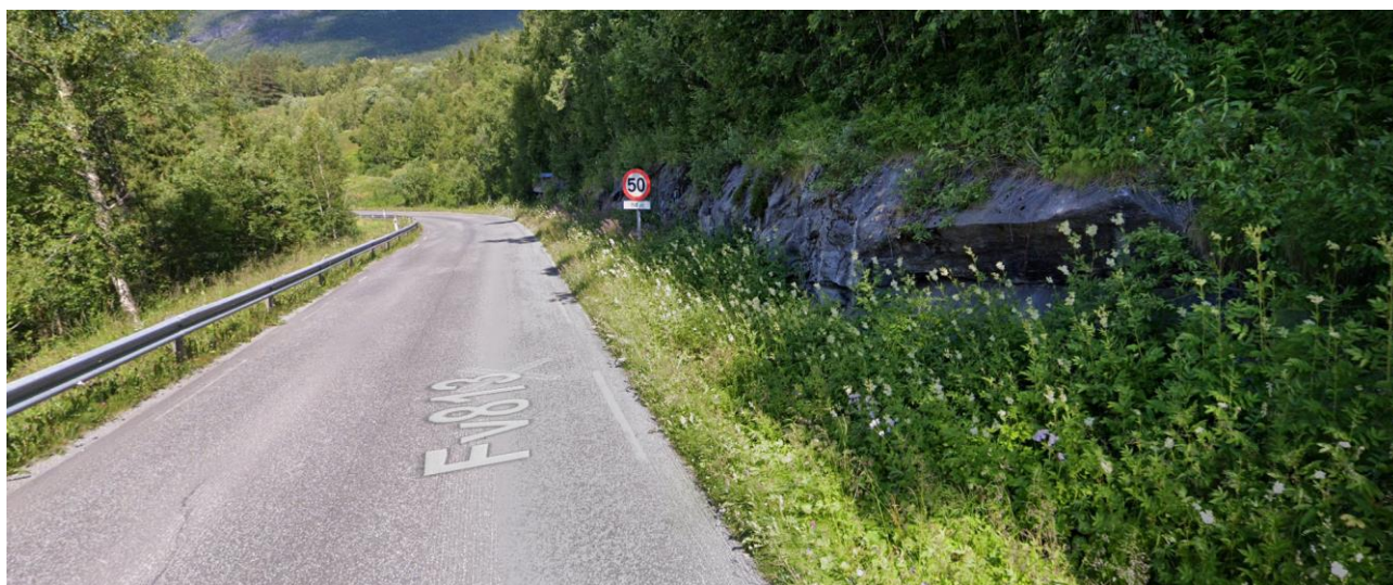
Figur 2-10: Bergskjæring, ca. P480.
